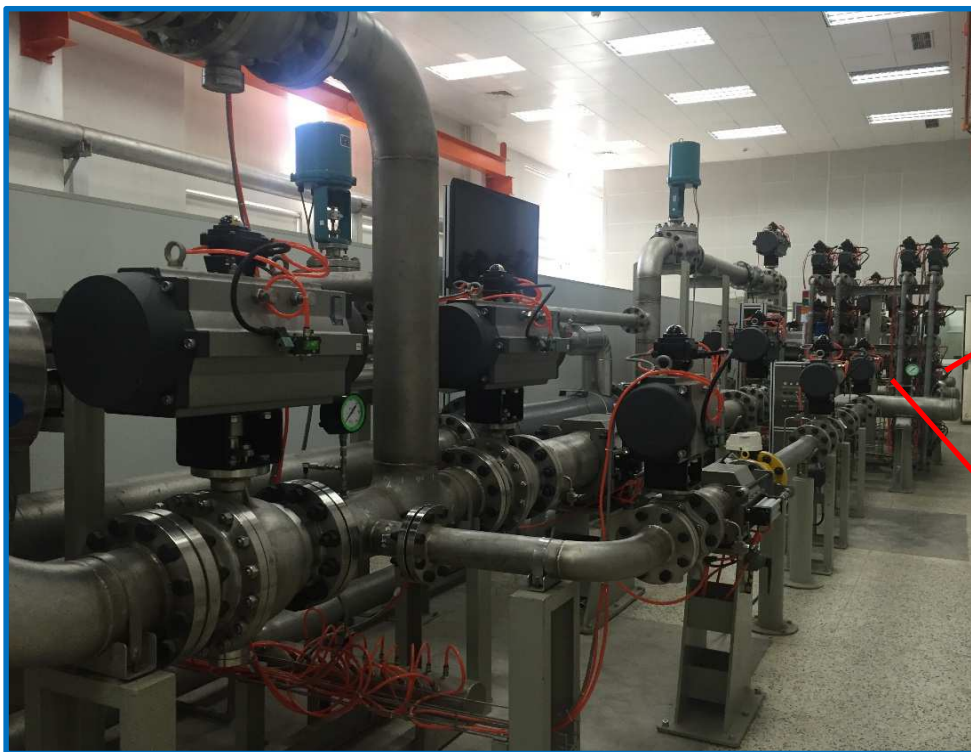
Overview of the facility
